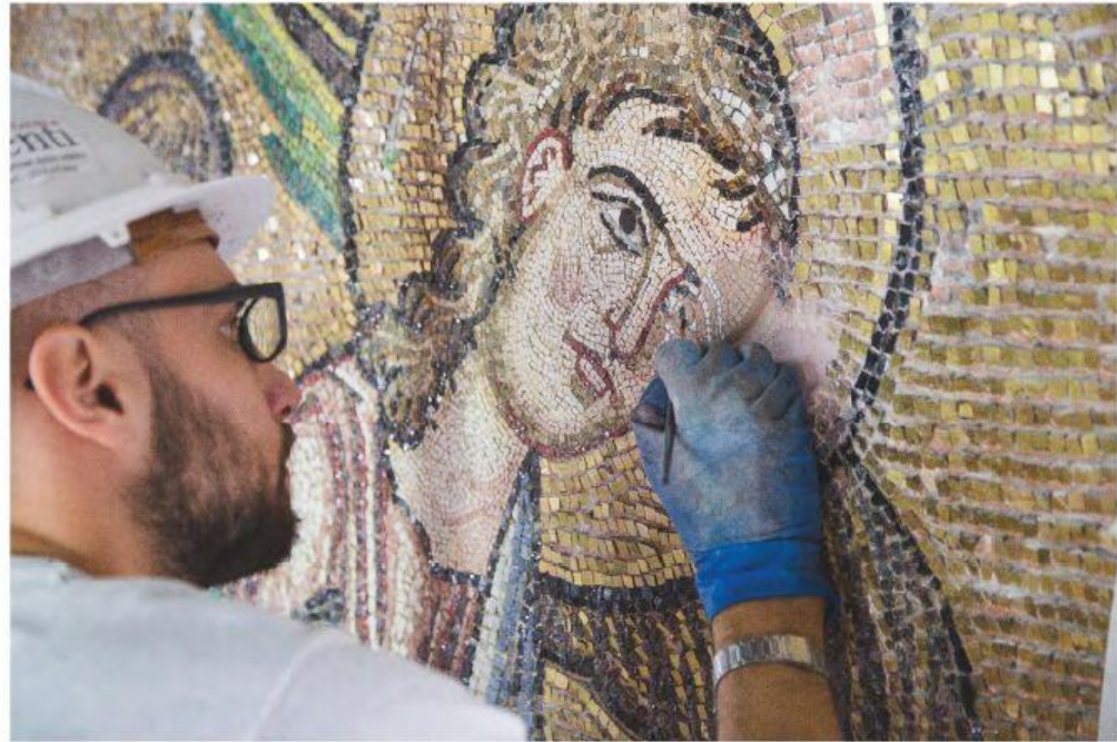
Restoration of the Nativity Church - Bethlehem
