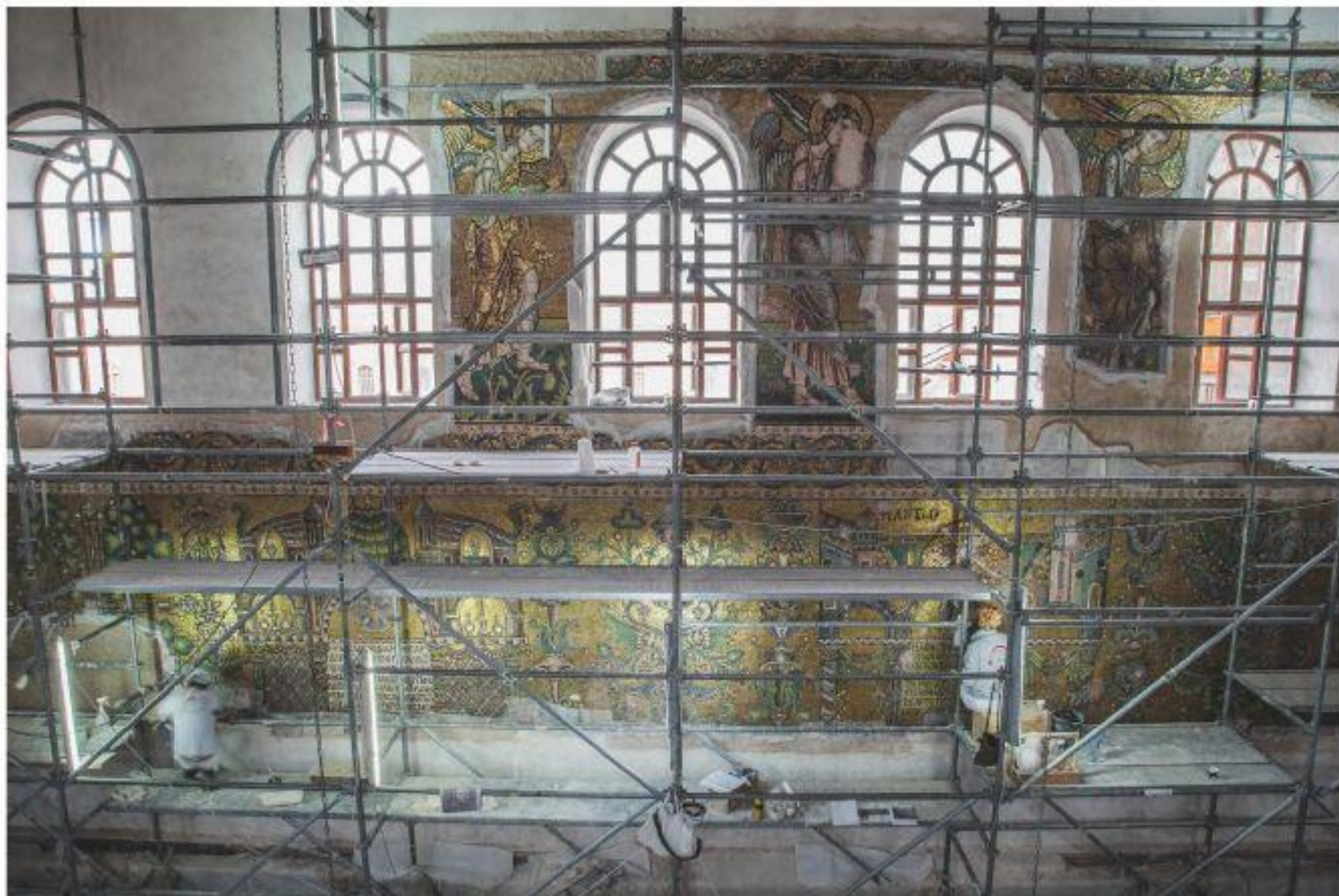
Restoration of the Nativity Church - Bethlehem
